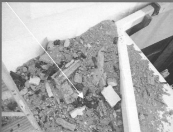
Again water infiltration thru roof, possibly 15 or more years ago, before any roof repairs.
