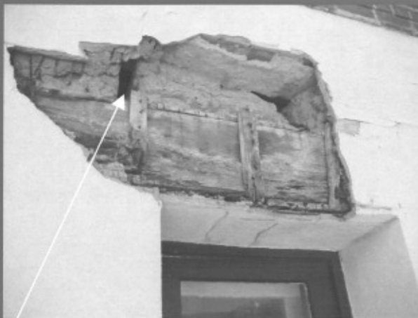
rotted wood joists
