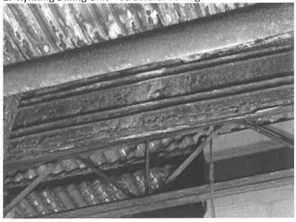
3. Rynning Detention Unit \_ Rusted Roof
