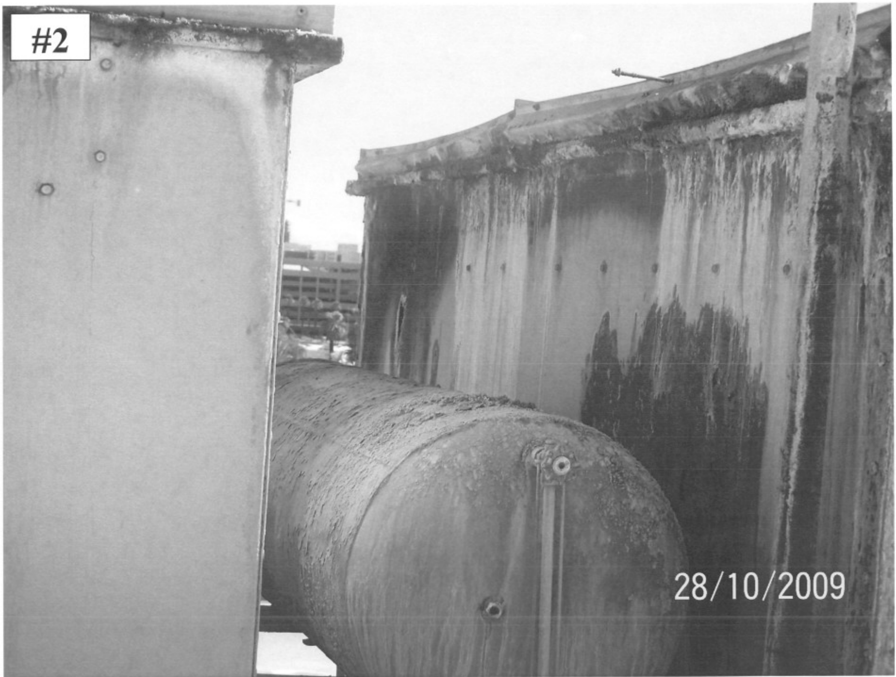
The picture is looking east at both cooling towers. The tank is an expansion for the building closed loop.
