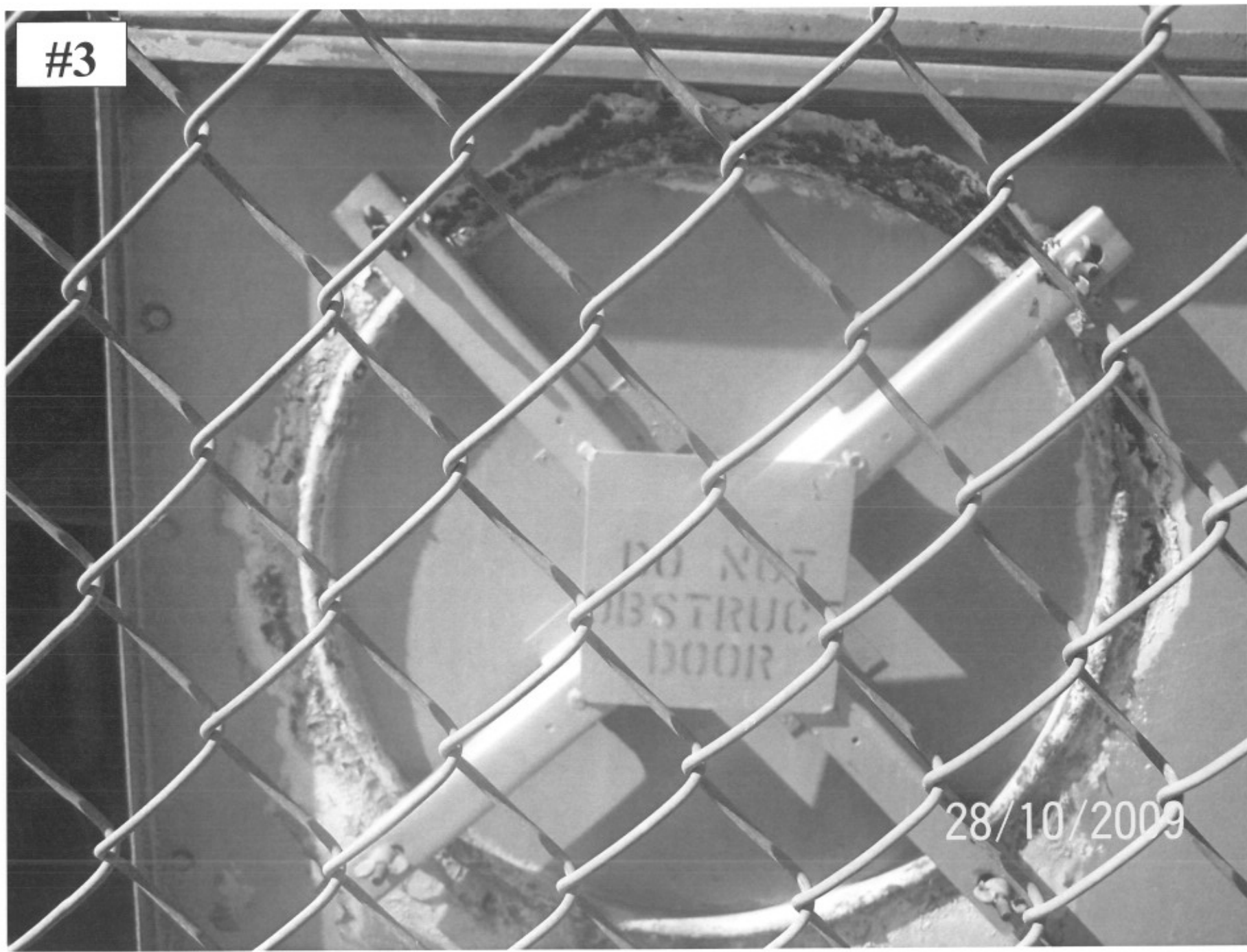
Door to enter wet section of tower.
